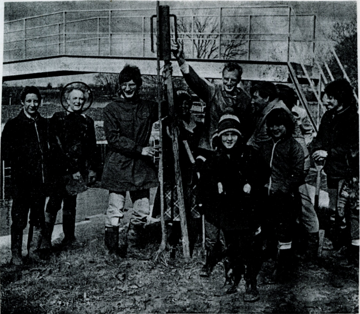
Villagers from Harvington planting trees at the newly-completed Robert Aickman lock at Harvington.
