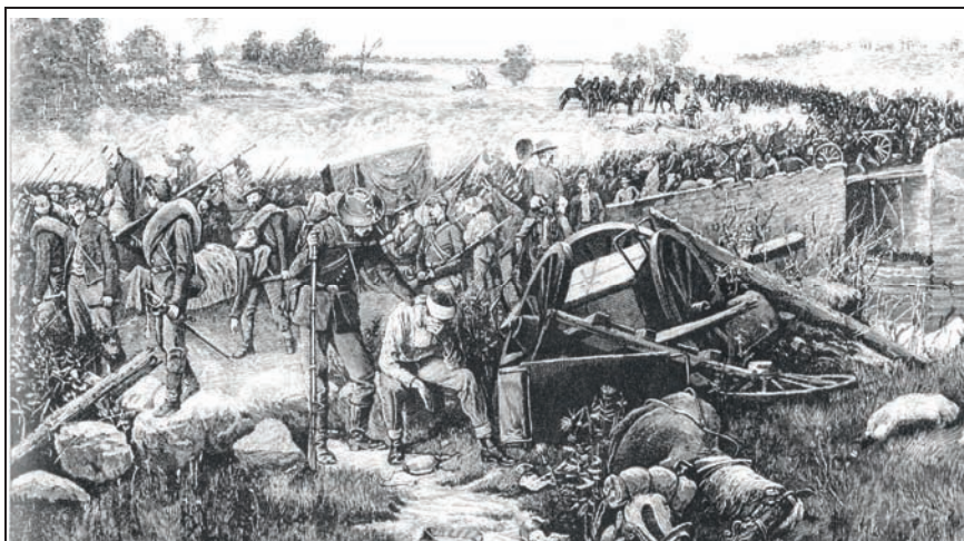
The retreat of the Union Army from the second battle of Bull Run, August 30, 1862. The wounded Barzetti / Shepherd would probably have been transported back over this bridge to hospital.
